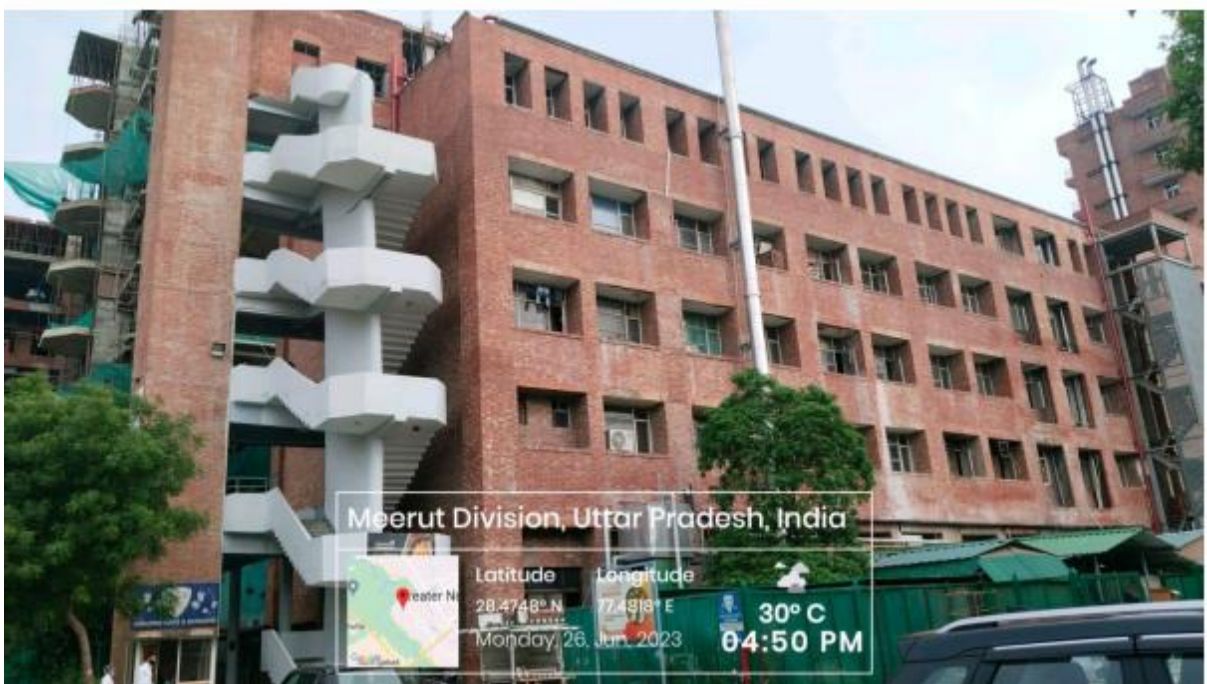
Fig 45 Nursing Staff Quarters Block 42
